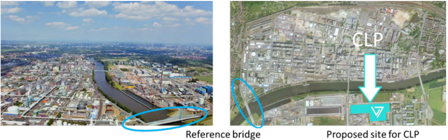
→ Figure 7: Höchst Chemical Plant and proposed site for the CLP
